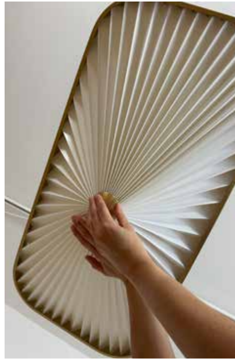
54. Place one hand on the shade as support while you unscrew the round brass button.
